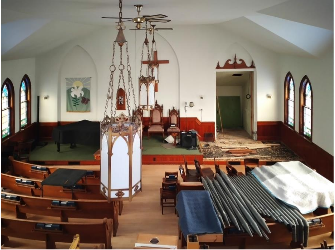
Here's the view of the chancel and the front of the nave from the space where the new organ pipes are now installed.
